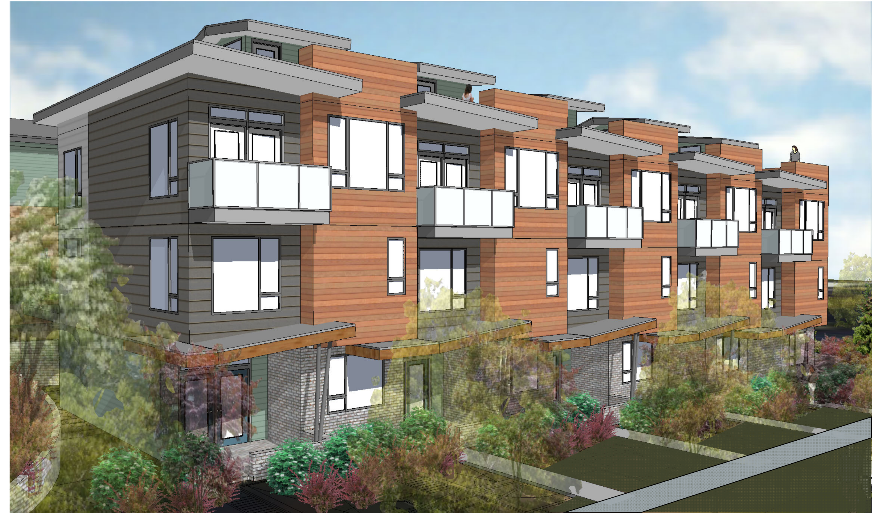
BUILDING 4 FROM DEPARTURE BAY ROAD
